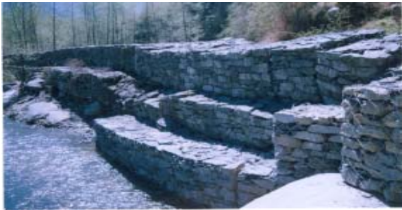
Checkdam constructed at Dhobi settlement
