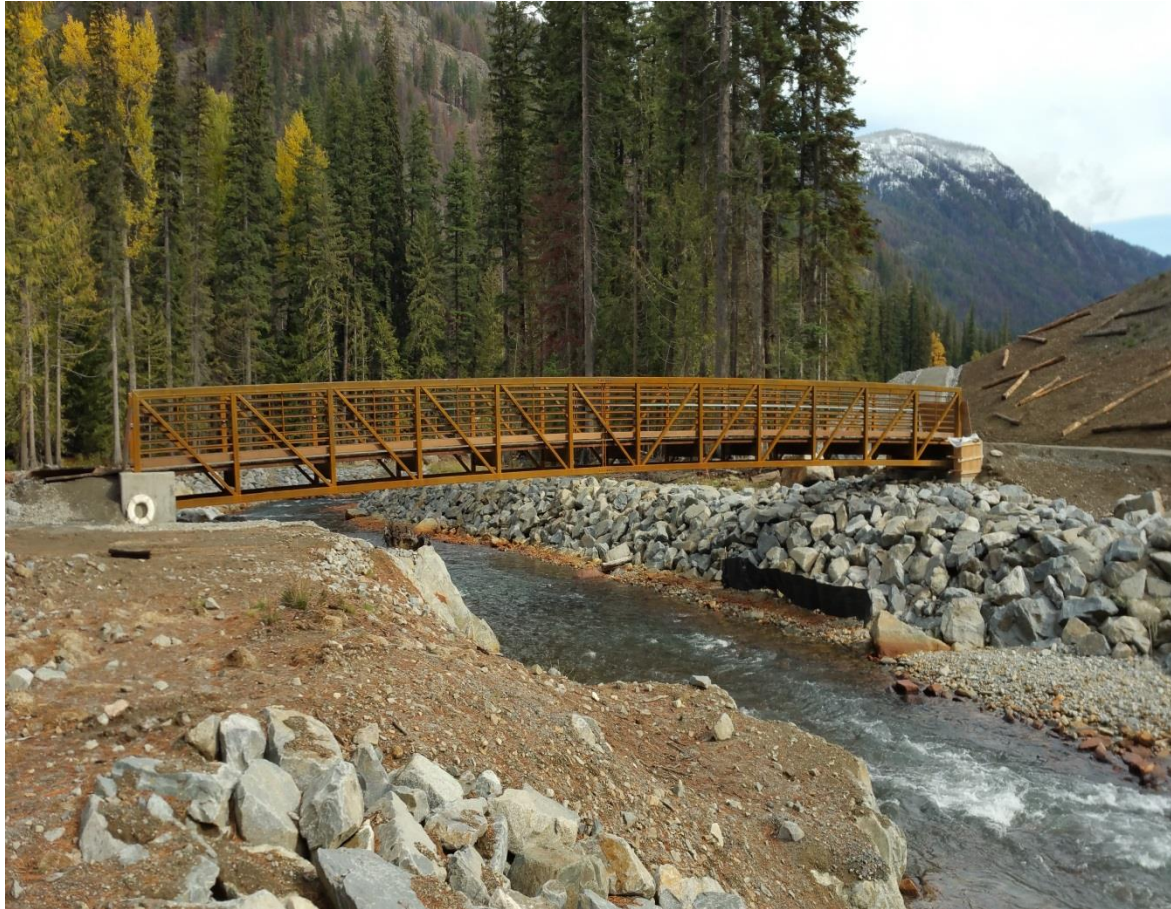
Holden Mine rehabilitation, Washington, USA Winner of the AEMA 2015 Environmental Excellence Award
