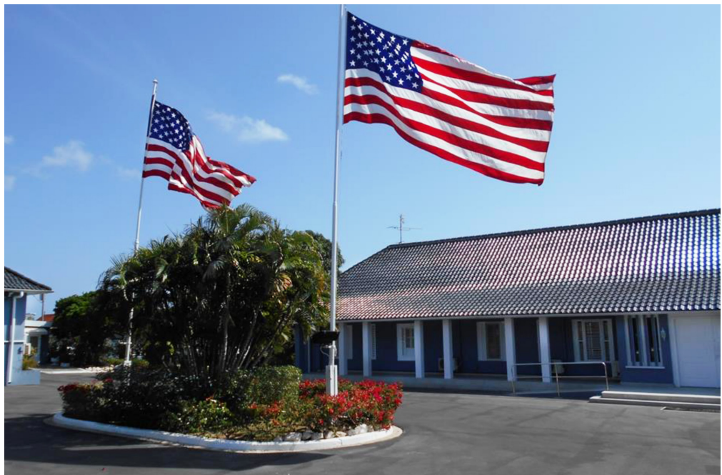
Consulate general compound in Willemstad, Curacao. (ISP-I-16-26A, 9/2016)
