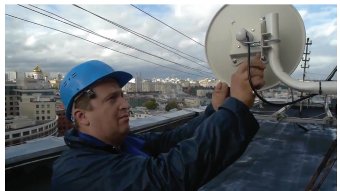
Enforta technician installs Ubiquiti product
