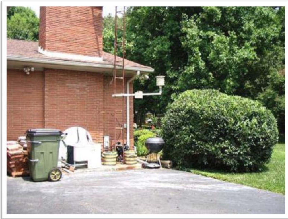
USHCN weather station at Hopkinsville, KY (Pielke et al., 2006). The station is sited too close to a building, too close to a large area of tarmac, and directly above a barbecue.
