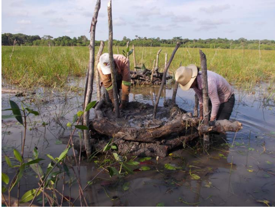
Illustration 5 Mangrove restoration to protect coastline in Alvarado, Veracruz (25 ha using “chinampas”) Source: (INECC, 2015)
