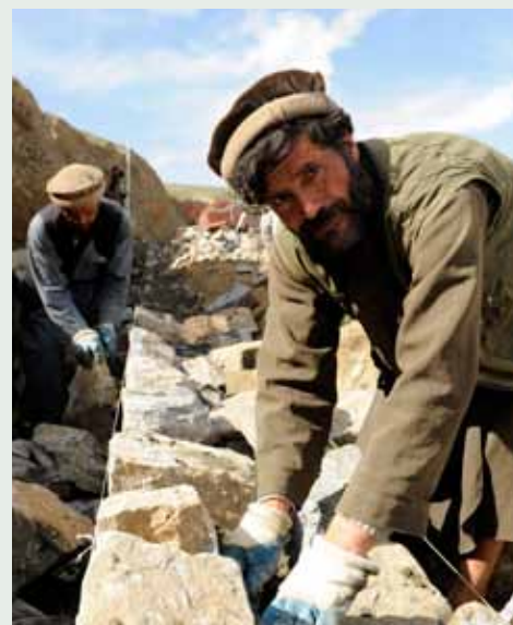
UNDP assists Afghanistan to restore infrastructure and provide much-needed jobs.
