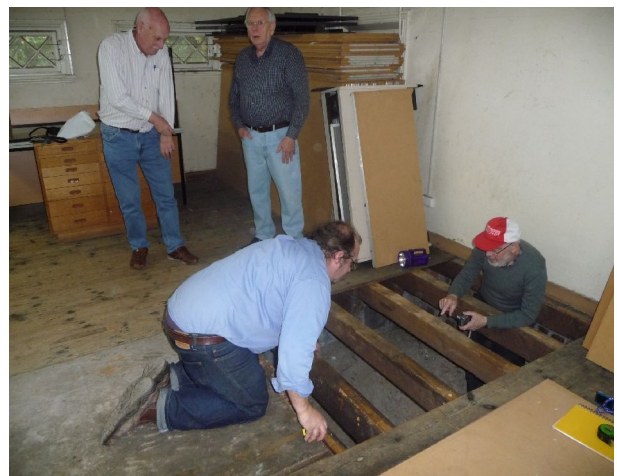
Inspecting under the floor in the GMT Chamber: Matthew Churchward of Museum Victoria is kneeling on the concreted top of the bluestone plinth. Dr Barry Clark is standing on the true ground, next to a deep test hole. Barry Cleland and George Littlewood are in the background.
