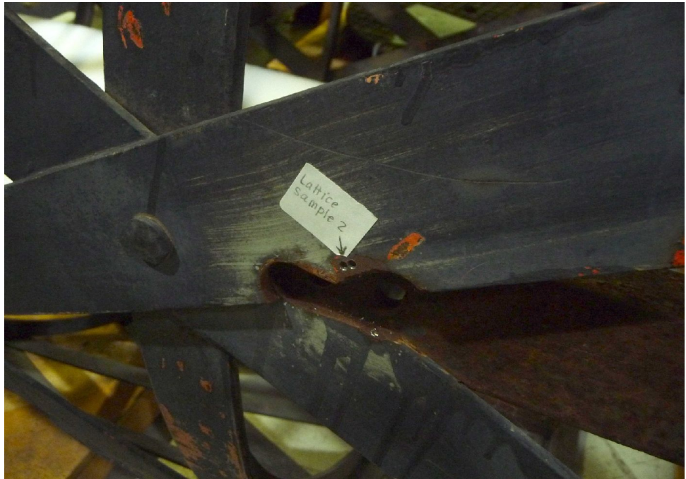
The lattice section of the GMT tube, showing two small drill holes from which a steel sample was taken for analysis.
