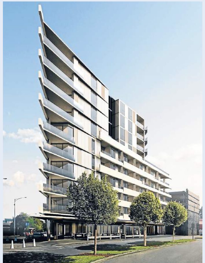
Above: The building's striking knife-edged design. Below: the north-facing residents' sky garden.
