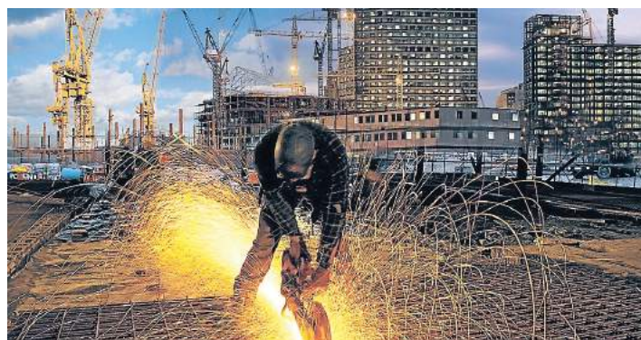
From top: Premier Tower, a spectacular 68-storey project at 134 Spencer Street; Melbourne's apartment-building boom is continuing.
