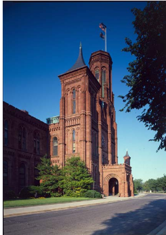
View of the Smithsonian Castle. Image from the National Park Service’s Historic American Buildings Survey. Image credit: Jack E. Boucher.
