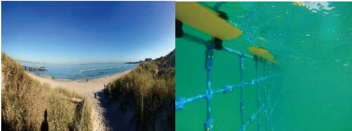
Figure 2-3 Eco Shark Barrier Net. Left: long view of Barrier at Coogee Beach, WA. Right: floats and barrier material. Source: Eco Shark Barrier Pty Ltd
