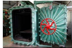
Autoclaves in Wharf precinct Map Ref D1 - Building A7
