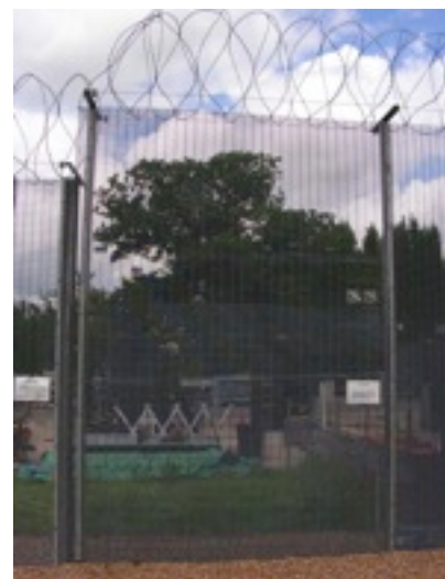
Picture 4: Class 4 security fencing
