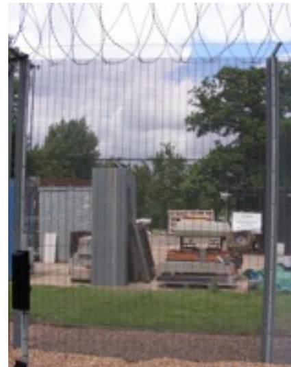
Picture 3: Class 3 security fencing
