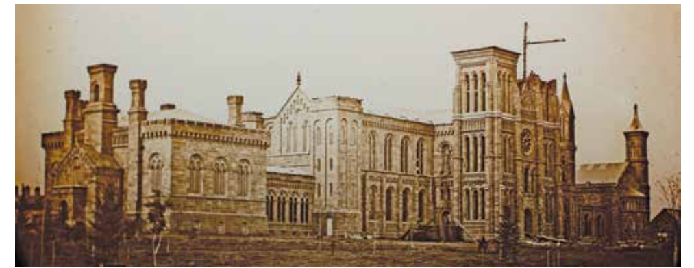
The earliest known photo of the Smithsonian Castle, taken in 1850, shows it still under construction. The rare halotype by Frederick and William Langenheim was a gift to the Smithsonian in 2015.
