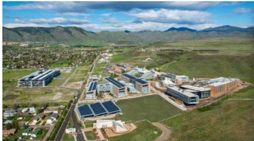
Photo by Dennis Schroeder, NREL 26954
