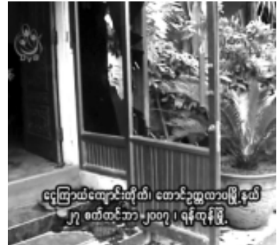
Smashed doors at Ngwekyaryan Monastery, September 27 (DVB)
