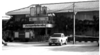
Kalasin District Police Station (Police website)
