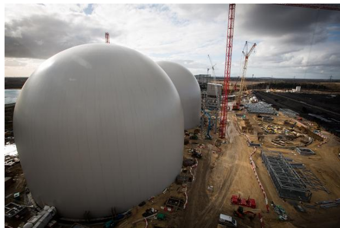
Photograph 2: New pellet storage facilities at Drax
