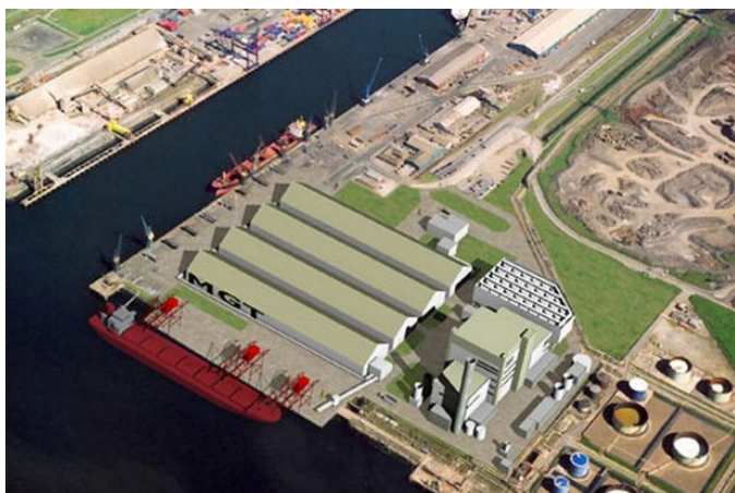
Photograph 1: Image of MGT Power's approved Teesside plant
