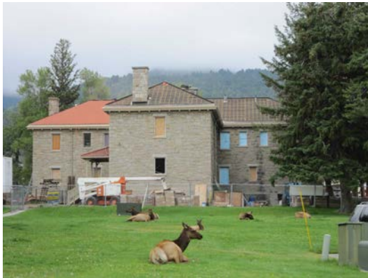
Exterior view of construction for the Yellowstone NP Albright Visitor Center
