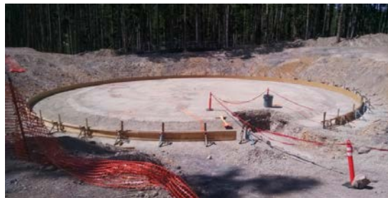
Foundation for a required storage tank associated with the Fishing Bridge Waterline
