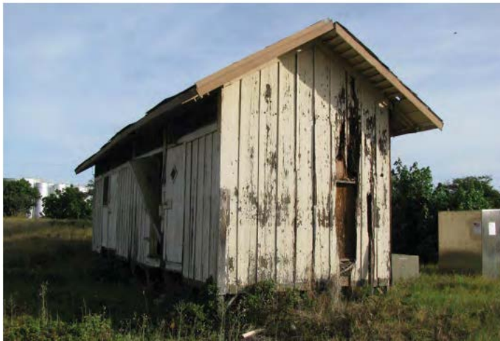
An old courthouse at Honouliuli NM; the park tells the history of internment, martial law, and the experience of prisoners in Hawaii during World War II.
