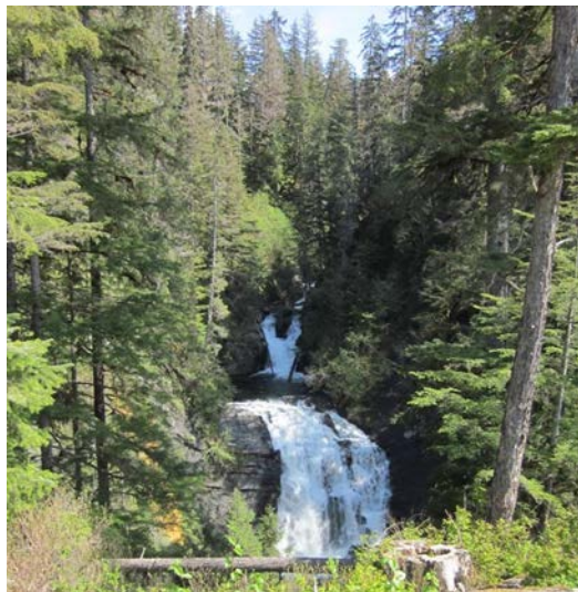
NPS is working with the new operator of the Falls Creek Hydropower Project, located near Glacier Bay National Park and Preserve, to implement license requirements to mitigate the project's impact on recreational and aesthetics resources.
