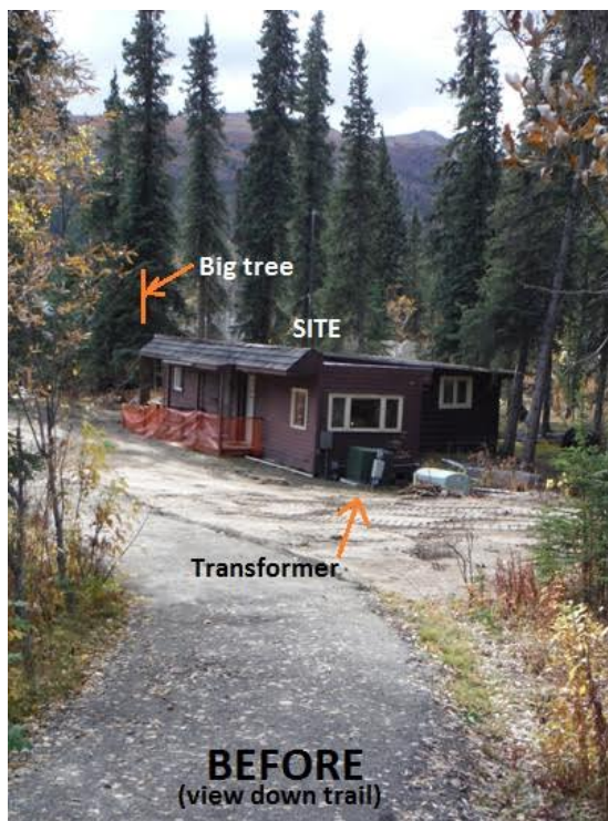
Denali NP&Pres obsolete former dispatch center
