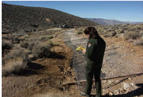
An open slope was closed with cable nets and wire mesh at Skidoo Gold Mine. Death Valley NP. California.
