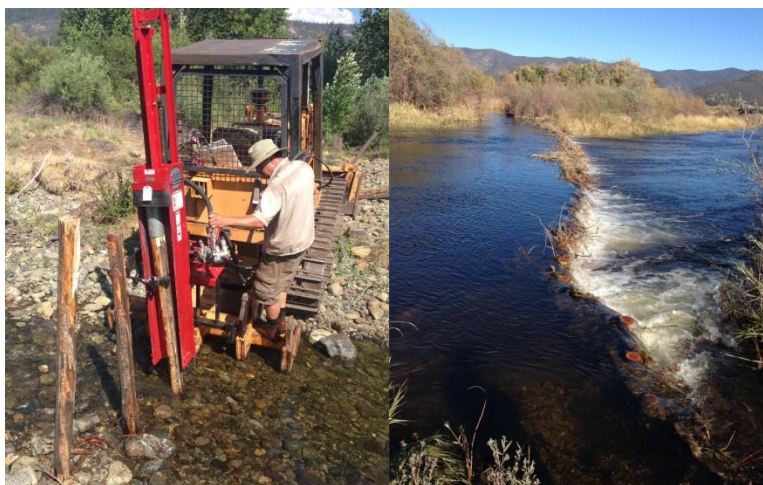
During restoration (left) and after restoration (right). Photo by Mark Cookson/USFWS
