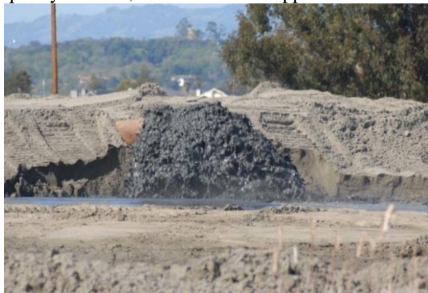
Sediment from the Port of Oakland used to restore the former Army Air Base at Hamilton Field back to wetland habitat Credit: Beth Huning
