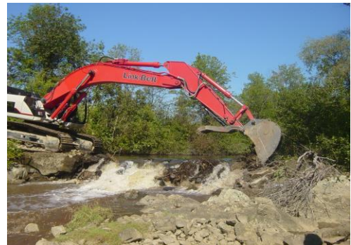
Goff Mill Brook Dam removal
