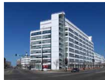
Nancy B. Jefferson Alternative School is housed in the Juvenile Detention Facility.
