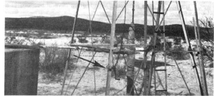
Windmill. Note windlass (arrow).
