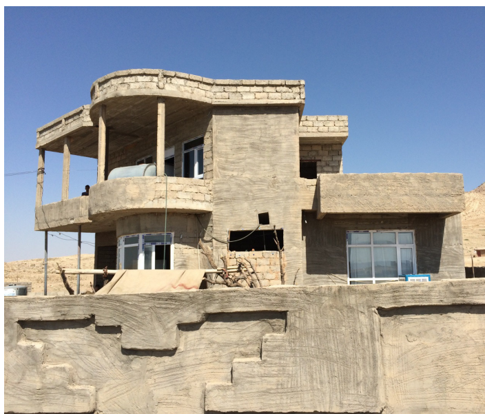
IDPs live in unfinished buildings like this one in Dohuk Governorate. Photo by OIG.
