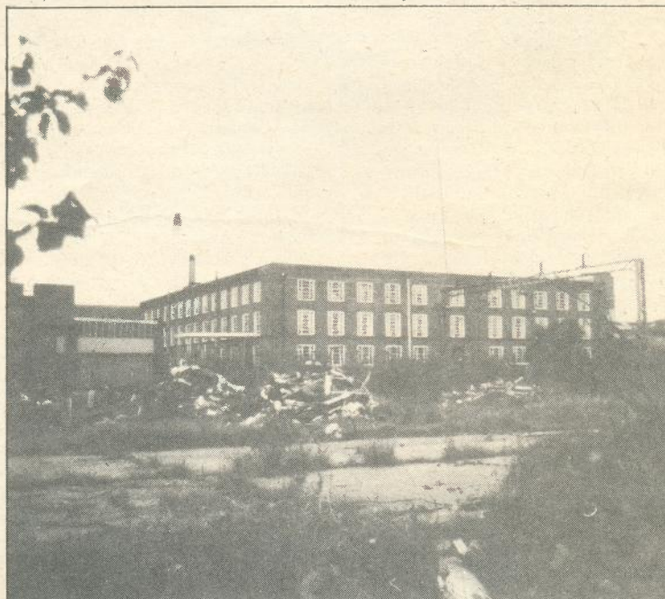
'Station Z': This wartime office block conceals a bomb shelter for central government in Harrow.
