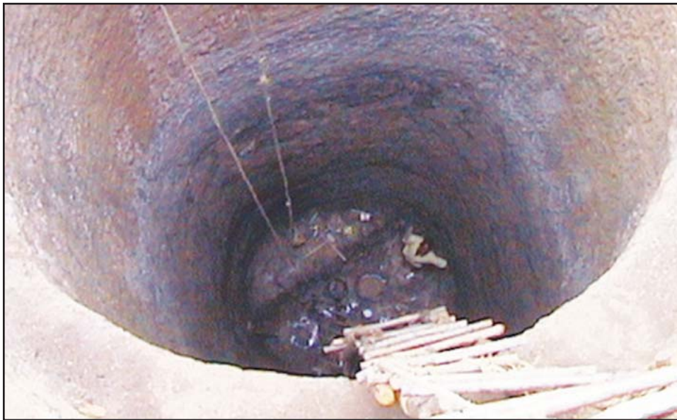
Picture 7: his well is currently being slowly excavated by two men. In many places in Kenya this construction takes months, if not years. When they are finished the seeping water is usually very low.
