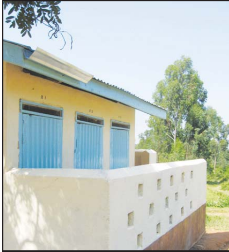
Picture 12: New toilets at school
