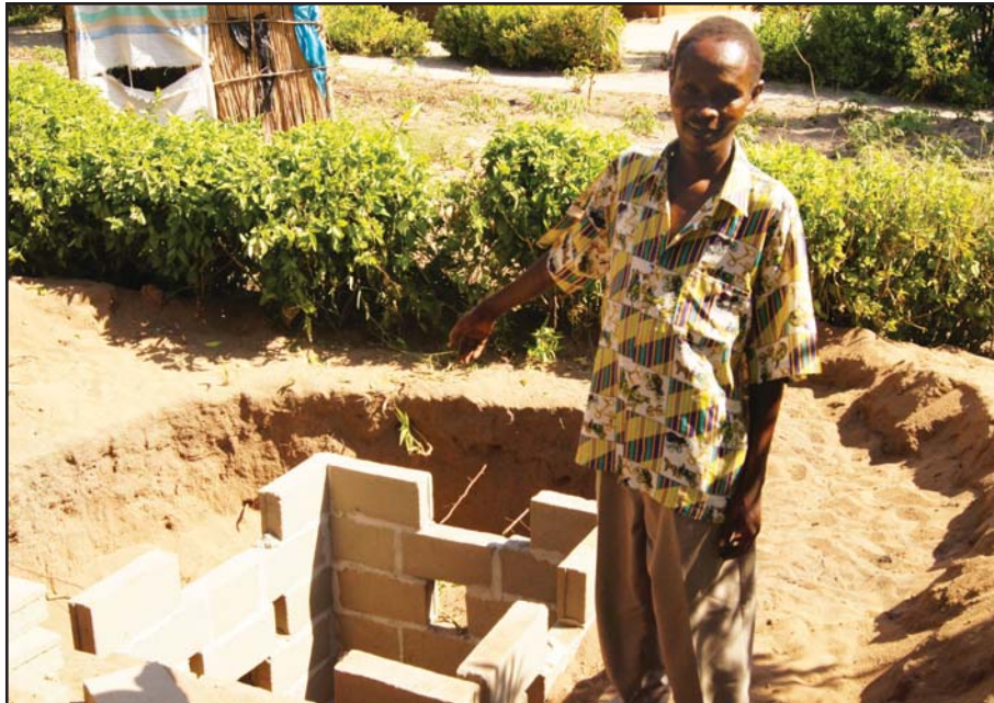
Constantino is showing the early work on the construction of his latrine. One of his goals is to build a latrine so his family can avoid diseases such as cholera and diarrhea. These diseases are often water-borne when contamination from feces occurs, mixing into their drinking water.
