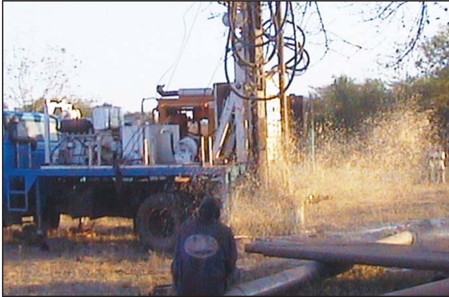
Water would come spraying out of the borehole when the operators blew out the sediment. The local villagers would dance and sing because they knew that they would be getting water shortly.
