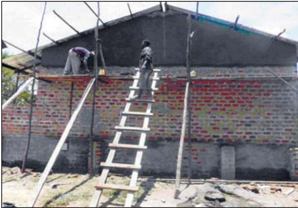
Picture 2: Parents help with Lufumbo school construction.
