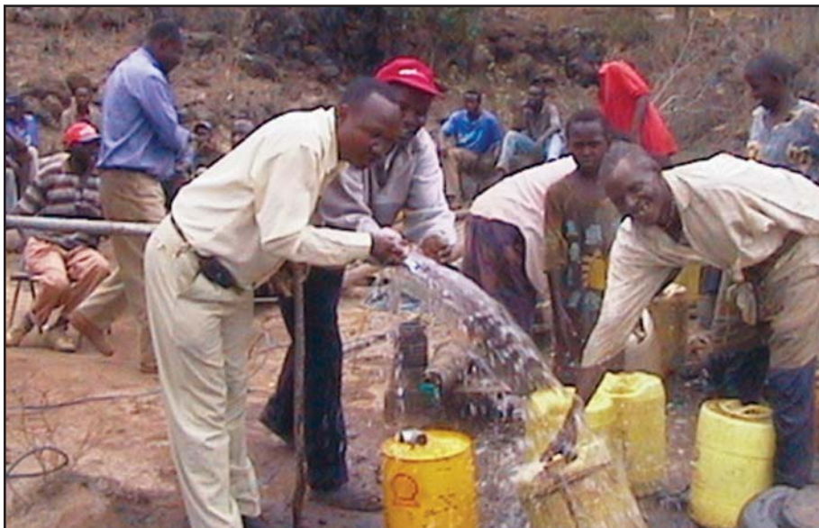
The water was pouring out from the well during the test pumping phase of the drilling operation. These men were overjoyed at the sight of all this water.
