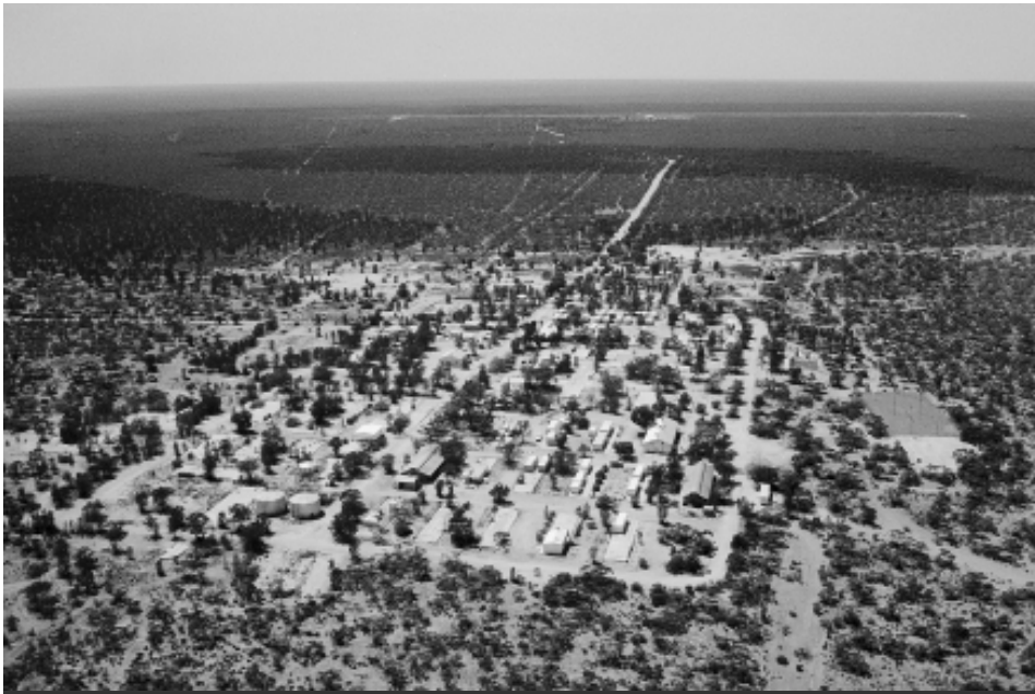
Figure 6.26 Maralinga village, looking east, airfield in background (circa 1998). Only about five of the original British buildings remain.
