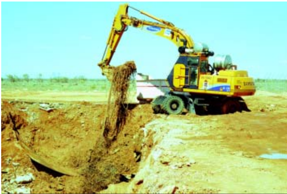
Figure 4.2 Class II modified excavator.
