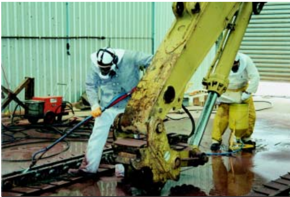
Figure 5.1 Fitters decontaminating caterpillar tracks.
