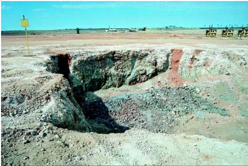
Figure 6.12 Exhumed pit 17 in central Taranaki prior to backfill.
