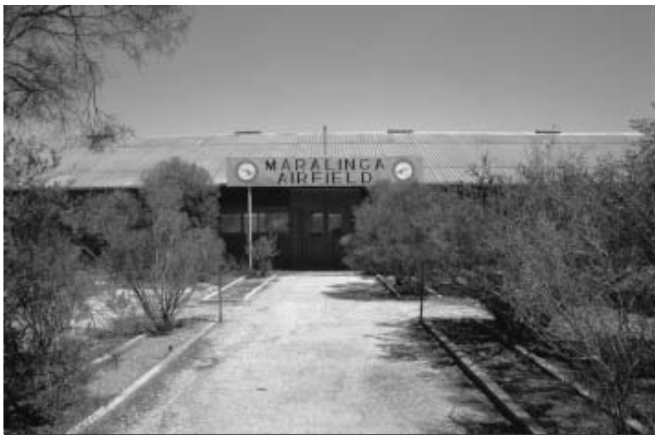
Figure 2.9 Old airfield building at Maralinga.
