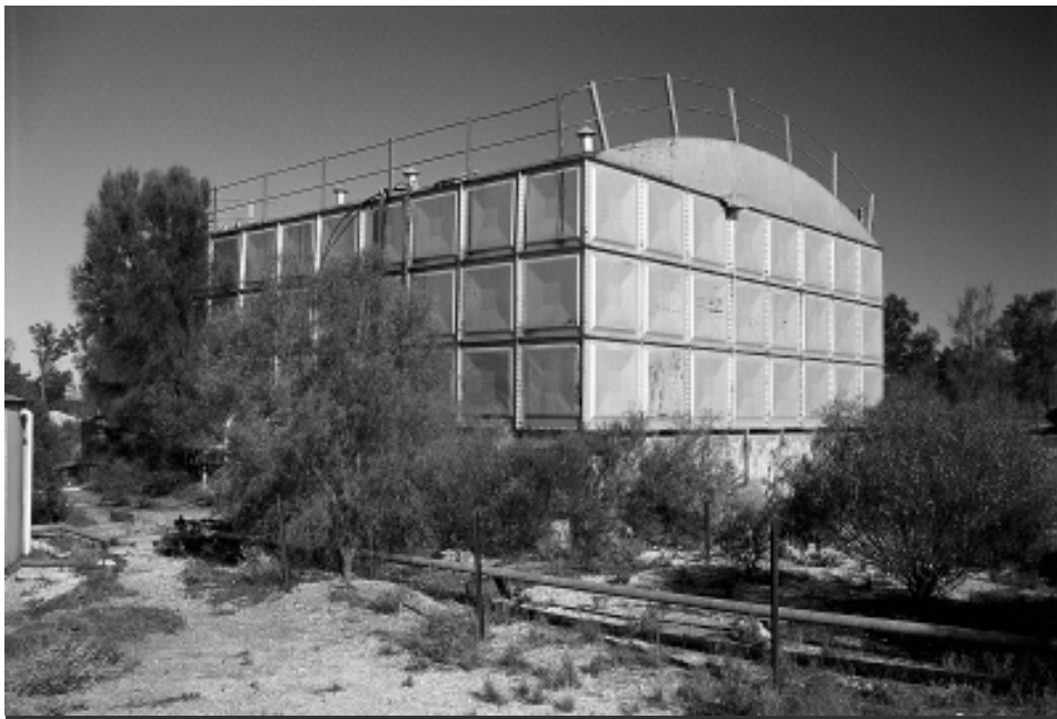
Figure 6.32 Halfway tank which stores rainwater collected from the airstrip.
