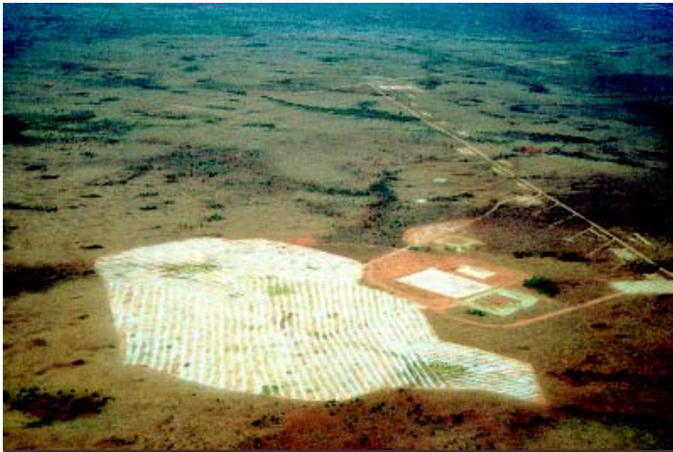
Figure 6.19 Aerial view of Wewak site after rehabilitation—with trench cap on right.
