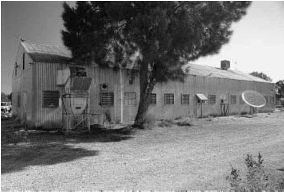
Figure 2.6 Rear of old hospital building.
