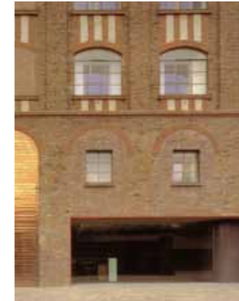
Figure 4.1.2p Clear address inserted into converted industrial building
