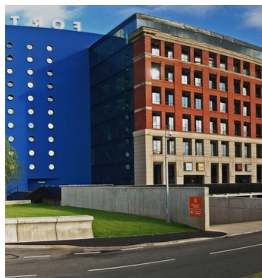
Figure 4.1.4e Fort Dunlop, Birmingham, Urban Splash. Adaptive reuse of large scale heritage buildings.
