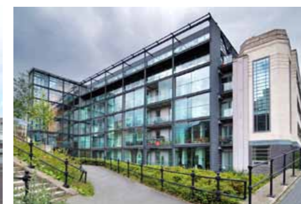
Figure 4.1.2v Mancuriam Way, Manchester, Urban Splash. Accommodating contemporary workspace requirements with heritage.
