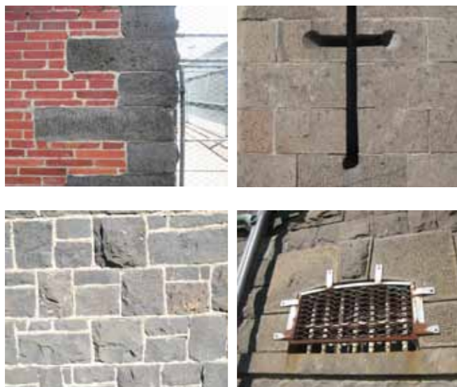
Figure 4.1.4p Bluestone Material Articulation
