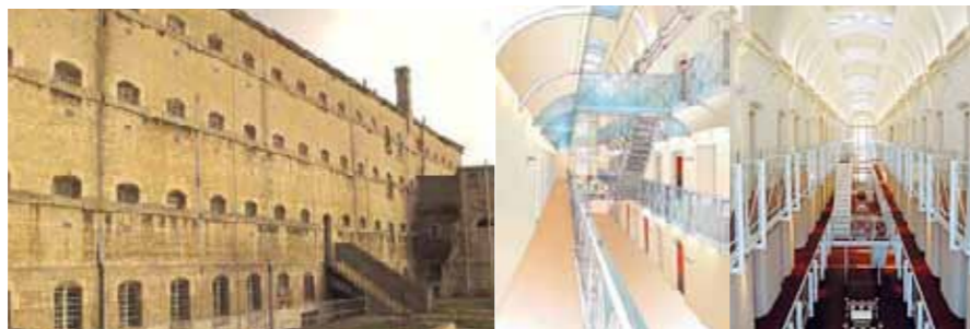
Figure 6 Images of the former prison building at Oxford Castle.
