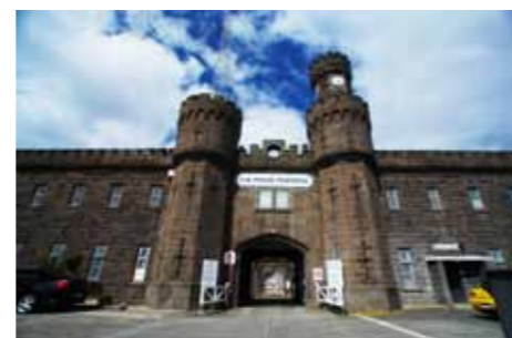
Figure 2.0c Former Administration Building
