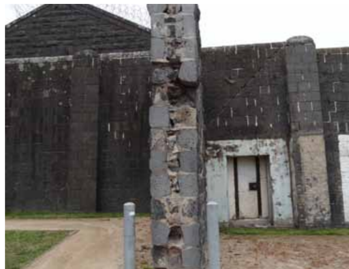
Current wall cut approaches already undertaken throughout the Pentridge area. We see these as not appropriate for Pentridge Piazza.
