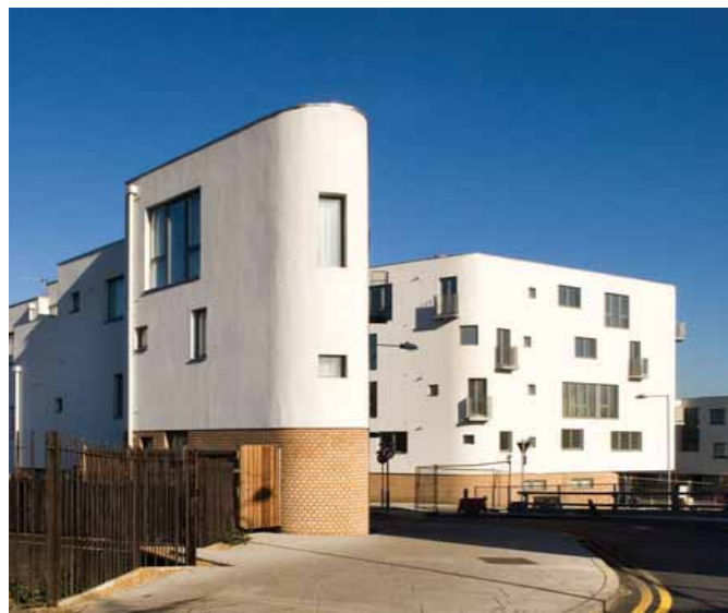
Figure 4.1.4a Allford Hall Monaghan Morris, Barking Town. Sculptural building forms and windows to reinforce wall edge.
