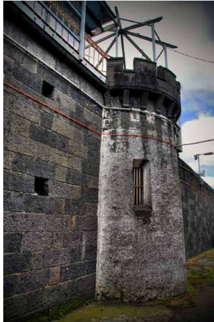
Heritage Wall fabric.
