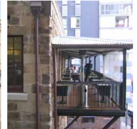
Figure 4.1.2r Adjacent 30 The Bond, Sydney.
