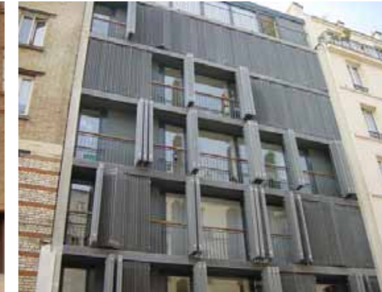
Figure 4.1.2q Herzoq de Meuron, Paris Layered and kinetic facade elements.
