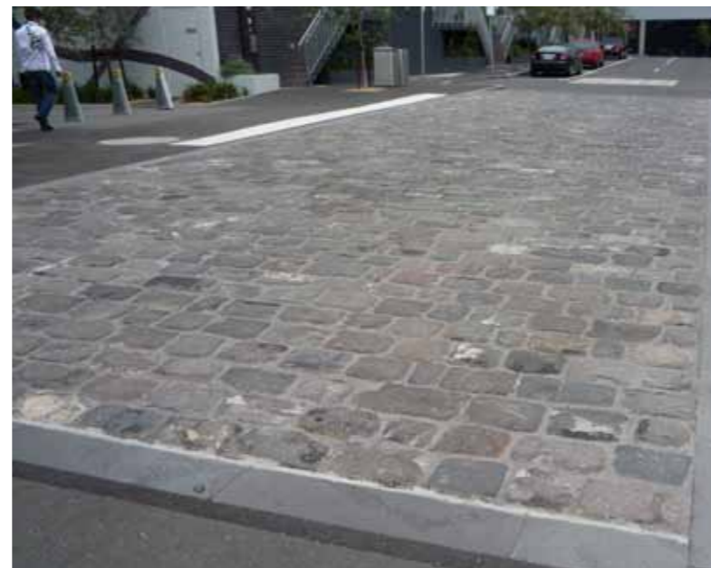
Example of proposed raised threshold (bluestone pavers)
