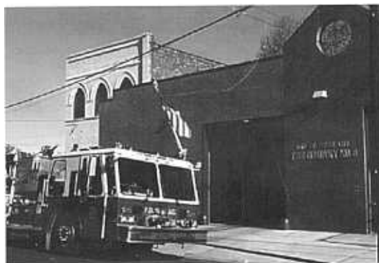
The new fire station replaced one that had been around since the early 1900s.
