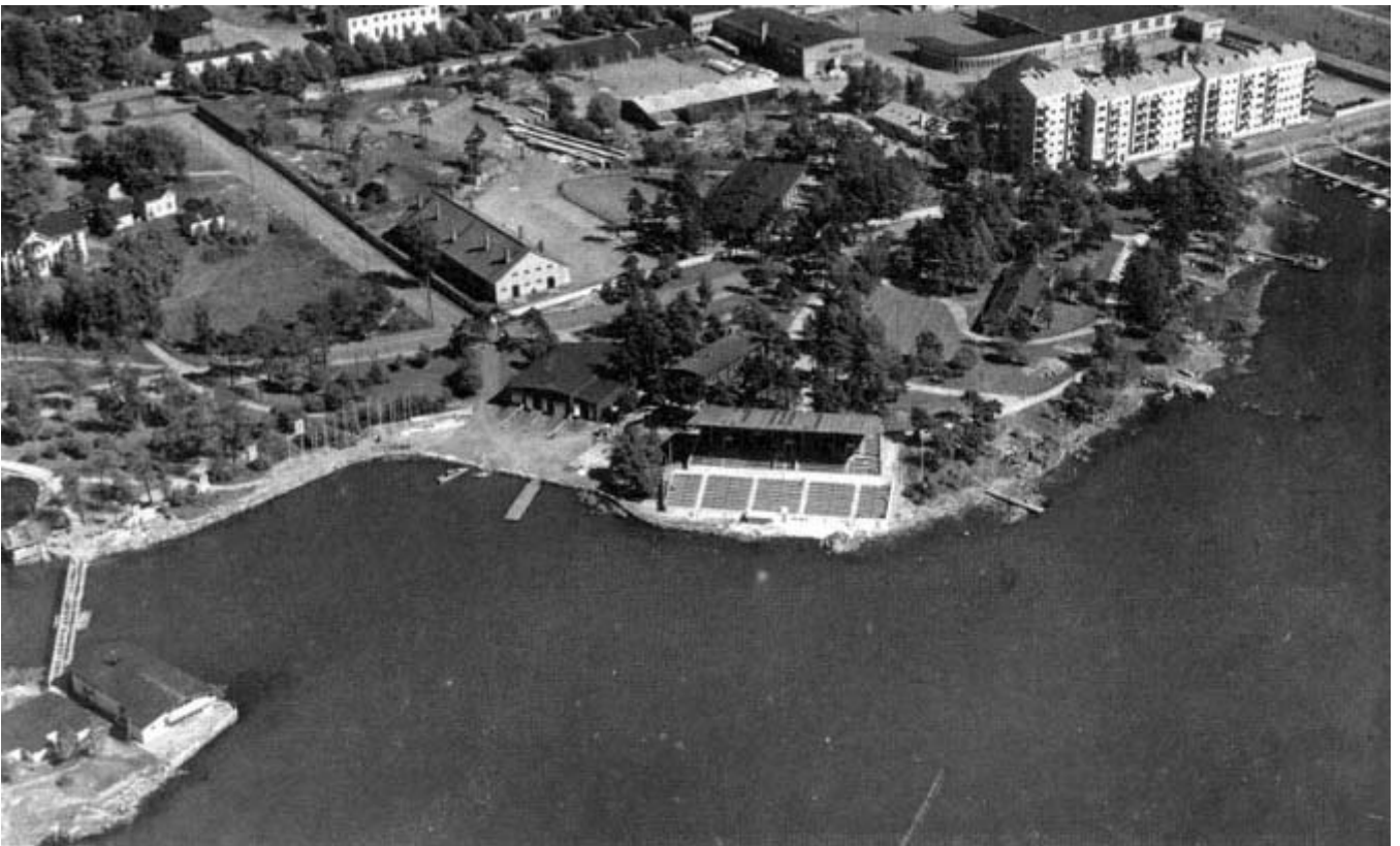
Air photo of the Taivallahti Canoeing Stadium.
