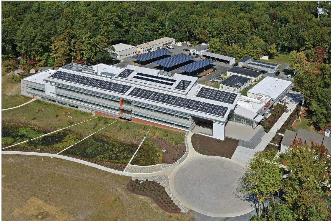
Smithsonian Environmental Research Center - Mathias Laboratory Building, LEED Platinum certified in FY 2015
