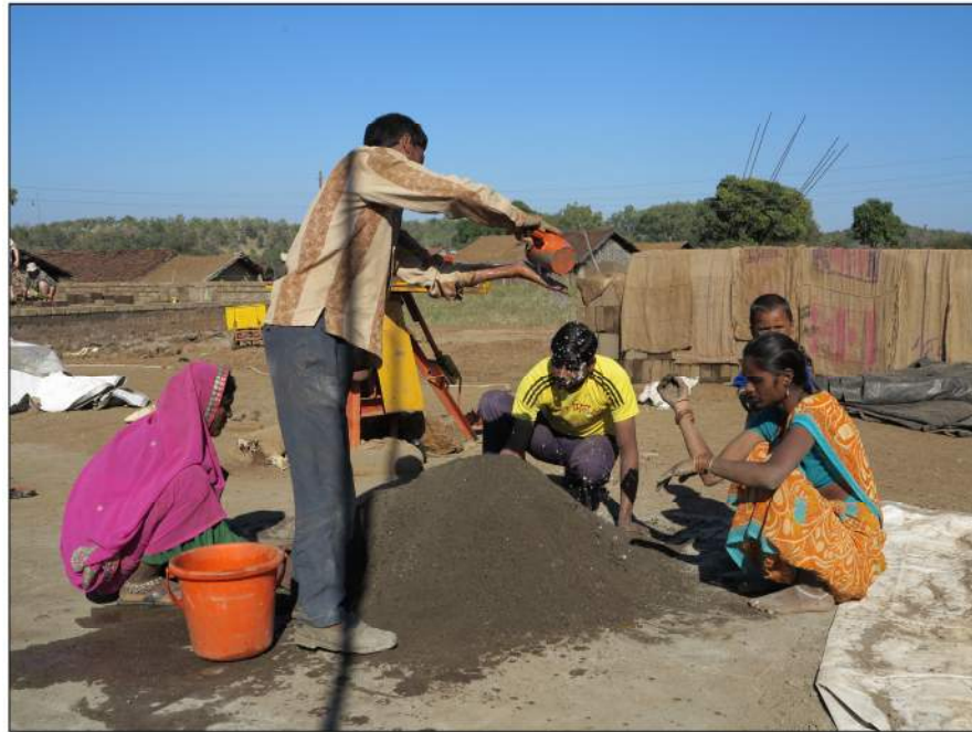
Photo 21: Mixing soil batch for CSEB production
