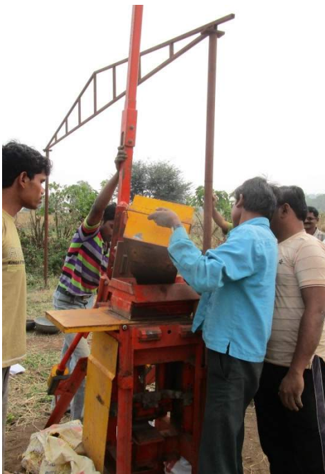
Fill block machine with soil, make block & test
