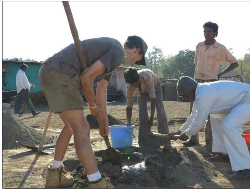
Photo 27: The teamwork continues
