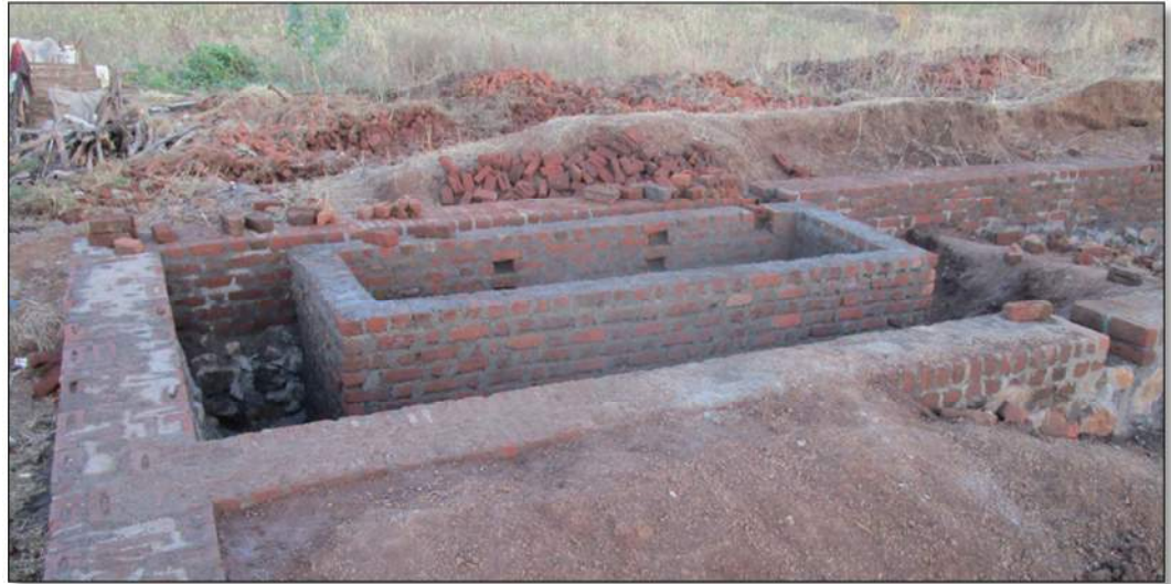
Photo 15: Septic and footings completed
