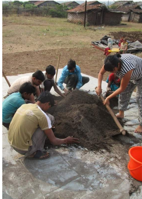
Measure & mix soil, sand, cement & water 6 times
