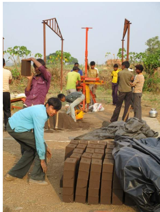
Stack for initial curing for 2 days under plastic
