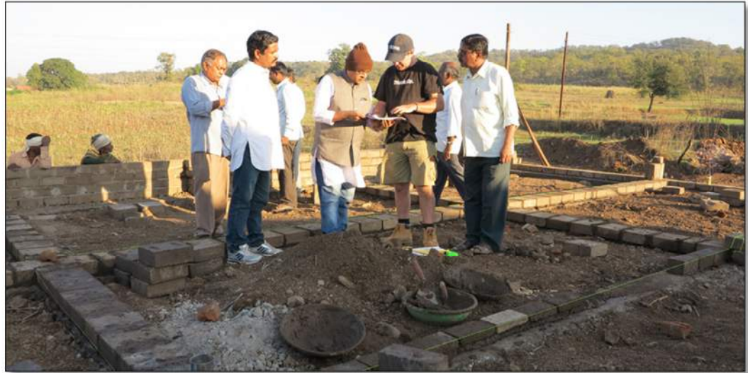
Photo 19: Finalise building layout and commence walls
