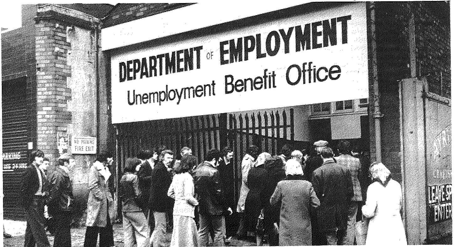
Dole office in Liverpool (Photo: John Sturrock, Report).
