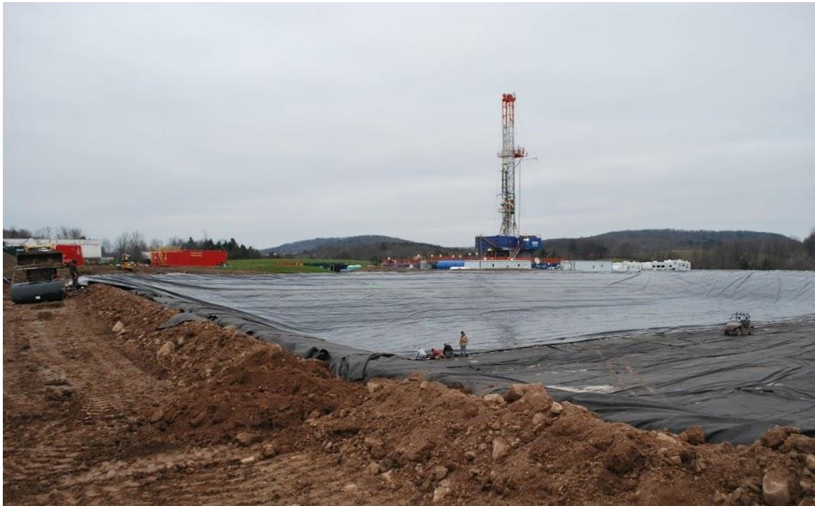
Centralized impoundment under construction in Pennsylvania. Photo by Frank Finan.
