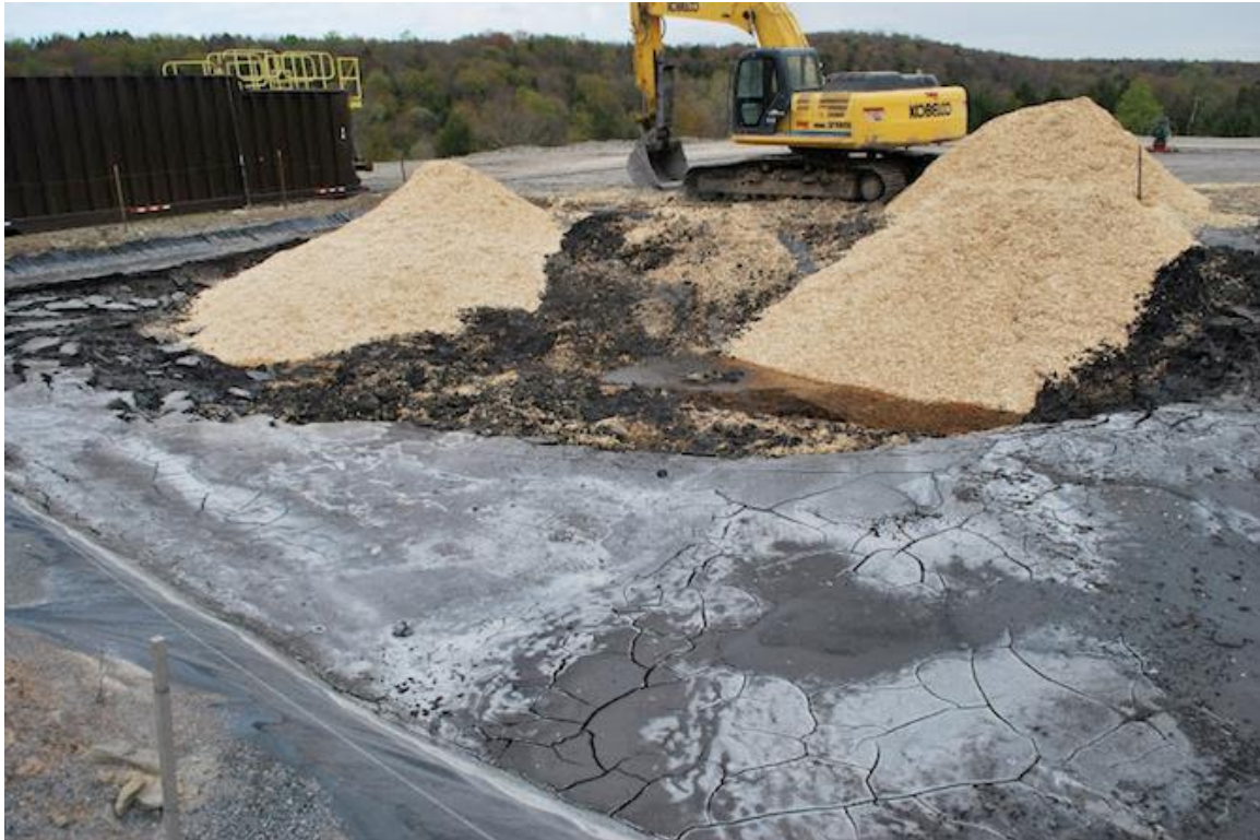
Sludge being blended with wood chips. Photo by US Geological Survey.
