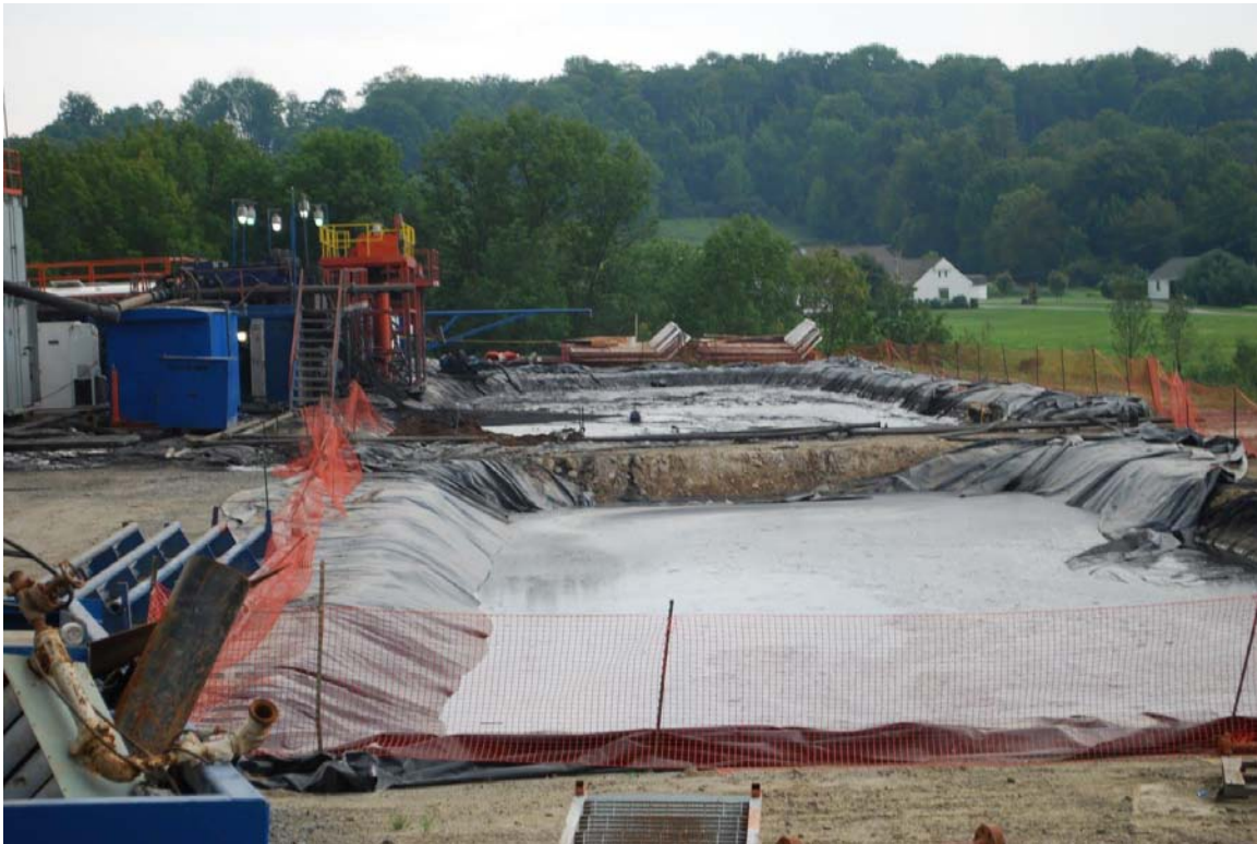
Waste pits under construction in Pennsylvania. Photo by Frank Finan.
