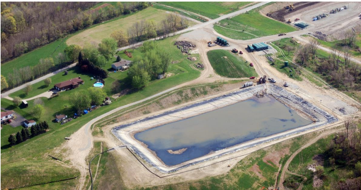
Centralized waste impoundment, Pennsylvania. Photo by Robert Donnan.
