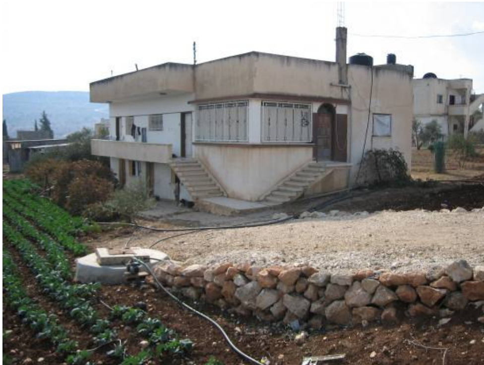
A rainwater harvesting scheme with pipe extending from the roof to a cistern, Jalboun
