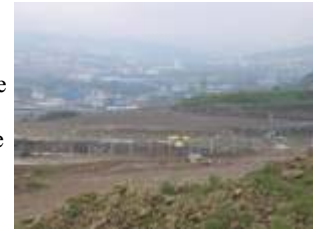
Parkwood Landfill site— home to another 650,000 tonnes of waste per year
