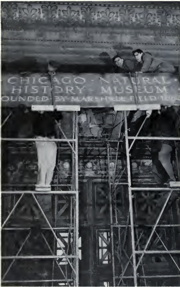
Museum workmen lower bronze nameplate from main entrance. After recasting, 700 pound plaque, bearing the new name, will be remounted.
