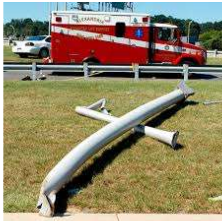
Figure F-2 – Downed light pole sections
