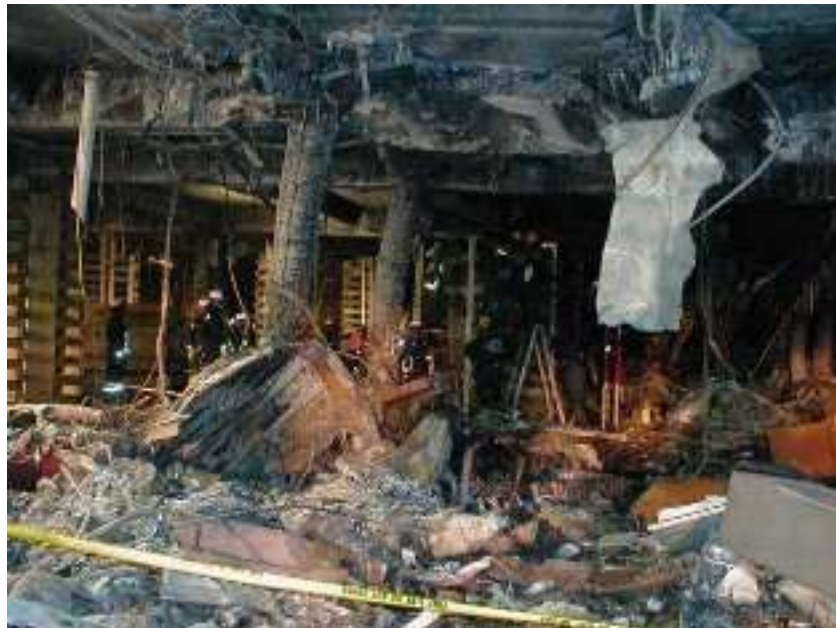
Figure G-4 Curved columns and aluminum metal
