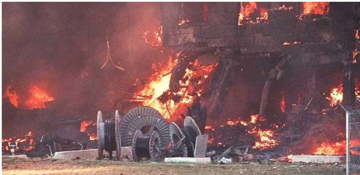
Figure F-10 Spools with fire ongoing
