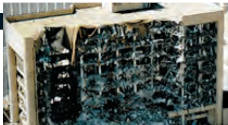
Murrah Federal Building
