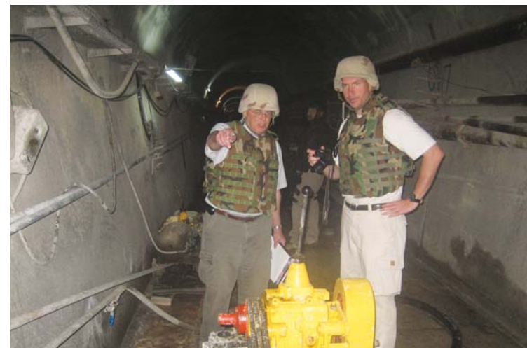
Members of SIGIR team inspect work at Mosul Dam.
