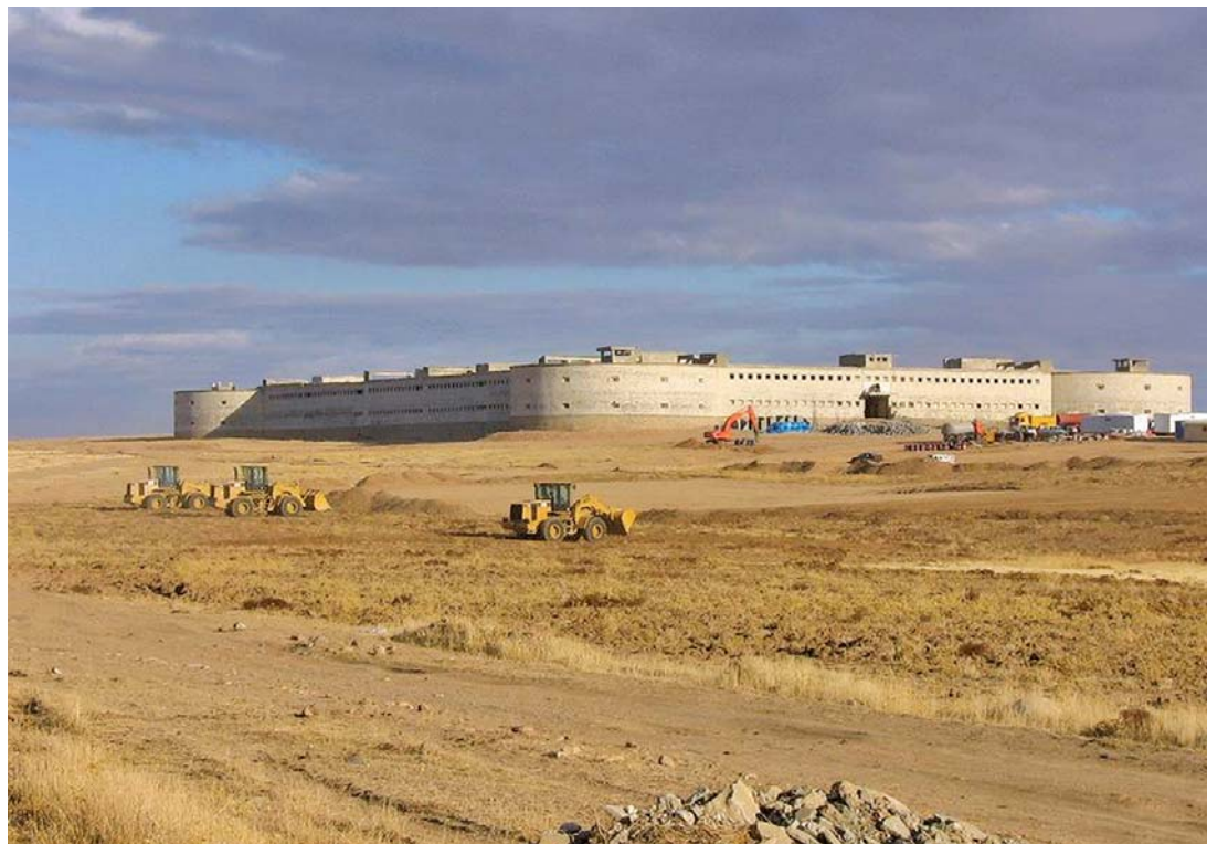
The $29 million Chamchamal Correctional Facility was completed in March 2009.
