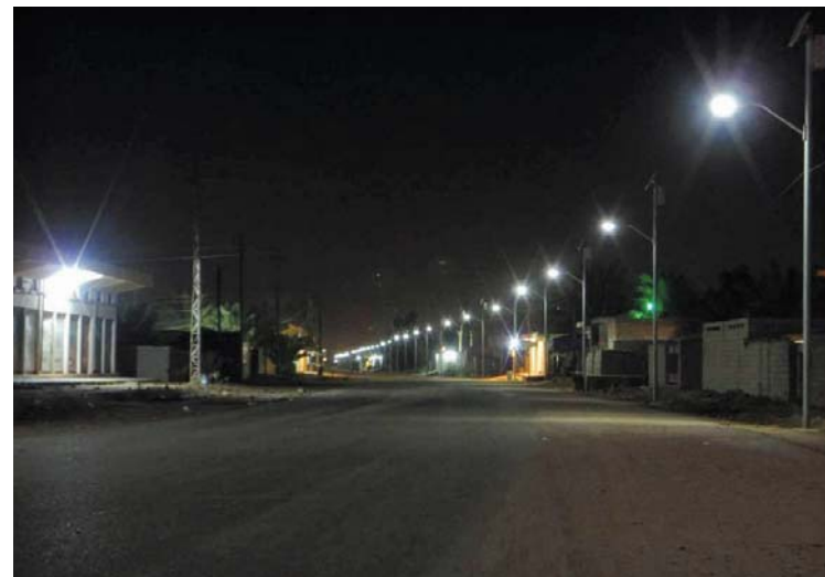
In a $10.2 million, CERP-funded project completed in three phases, USACE installed 1,200 solar-powered street lights along 35 kilometers of roadway in and around Falluja. (USACE photo)
