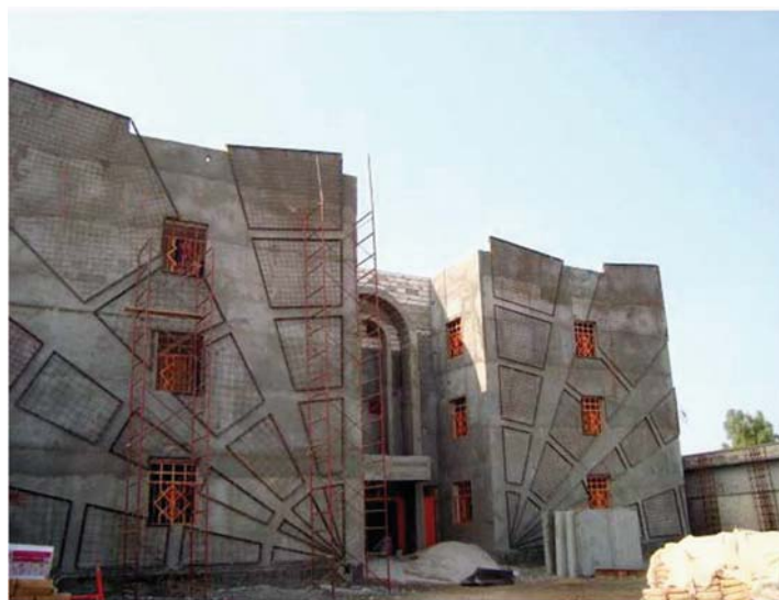
The U.S.-constructed Shatt al-Arab Courthouse in Basrah province was completed in June 2009. (OPA photo)
