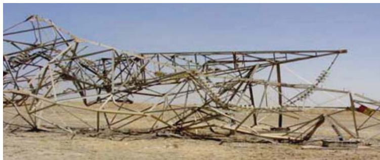
Primarily because of looting and sabotage, almost 1,000 electrical towers were destroyed and control systems were damaged, causing Baghdad and beyond to experience frequent blackouts in mid-2003. (Bechtel photo)
