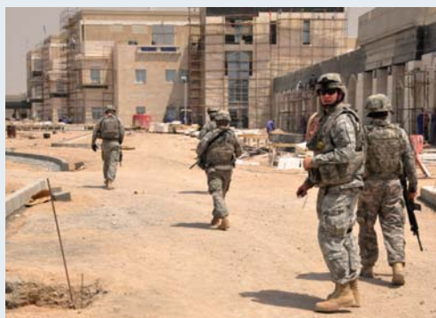
U.S. soldiers look over the grounds of the Basrah Children's Hospital under construction in May 2009. (U.S. Army photo)
