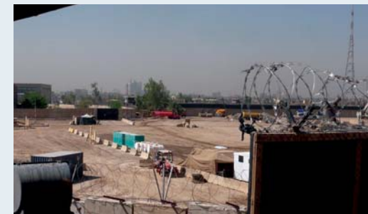
INL spent more than $100 million renovating facilities at former Forward Operating Base Shield, which was to be the main PDP basing area, before terminating construction, removing all advisors from the site, and turning the property over to the GOI.
