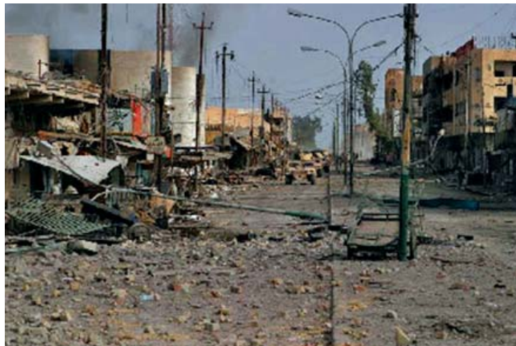
Falluja had become a lawless, chaotic place by mid-2004, with insurgents in complete control of the city, yet in June of that year the CPA awarded a $28.6 million task order calling for the completion of a new sewerage network by February 2006. (USACE photo)
