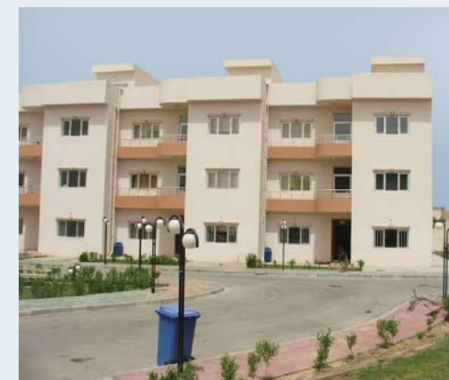
The quality of work at the U.S.-funded project in Erbil was the best SIGIR ever observed.
