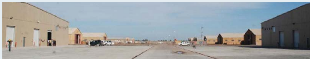
The Depot Distribution Central Operation storage facilities at Camp Taji was completed in November 2010. (USACE photo)
