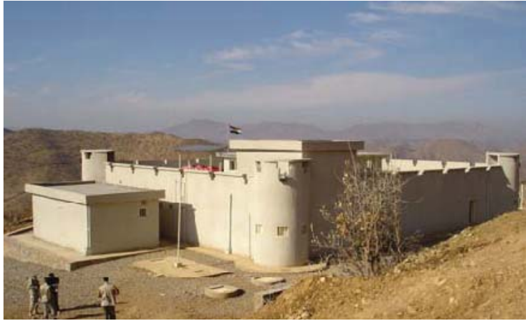
SIGIR conducted project surveys of 21 border forts located along the Iraq-Iran border.
