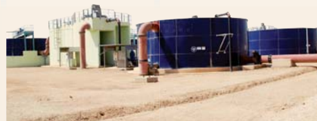
After: Completed WWTP in 2011
