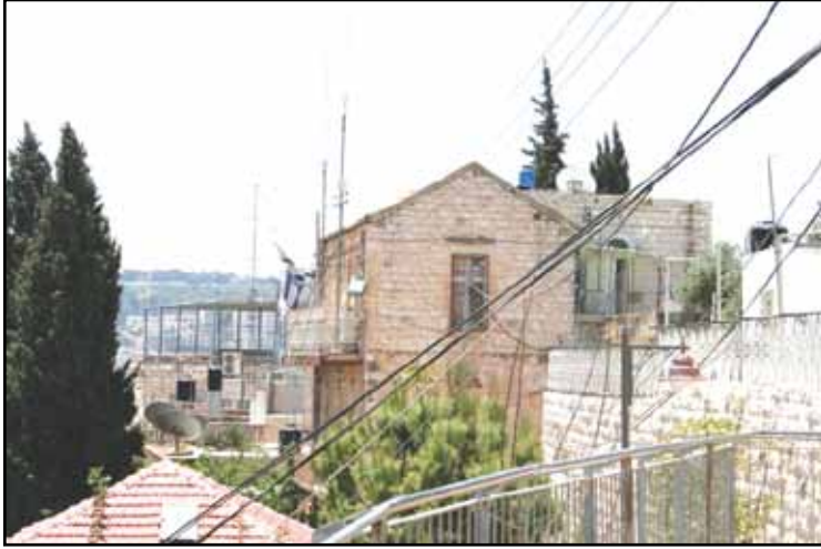
The Abbasi House. (Photo by: Emek Shaveh).
