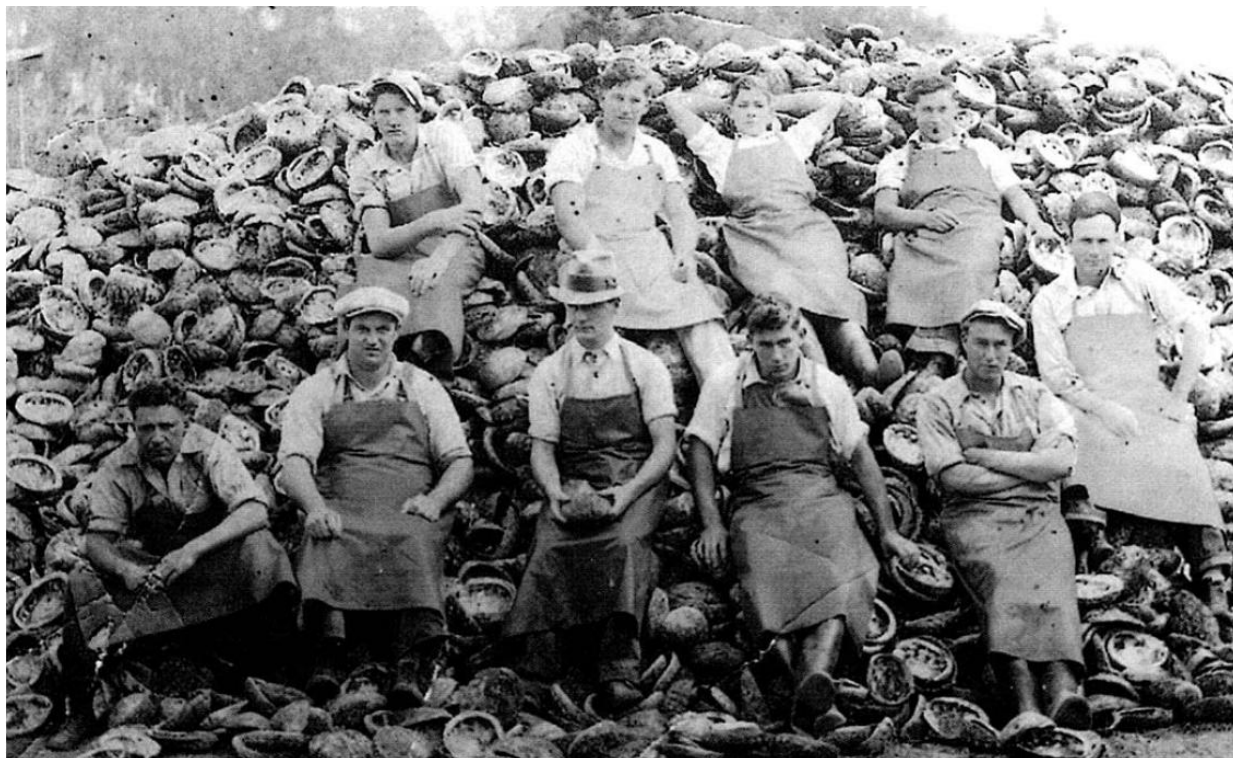
Figure 7: Pierce Brothers abalone processing plant, ca. 1933. Photo by Pat Hathaway, Source: Rogers-Bennett et al. 2002.
