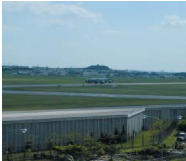
Sound insulation walls installed at the north side of Kadena Air Base as one of the Noise Reduction Initiatives agreed upon in the SACO final report. (at the front of the photograph)
