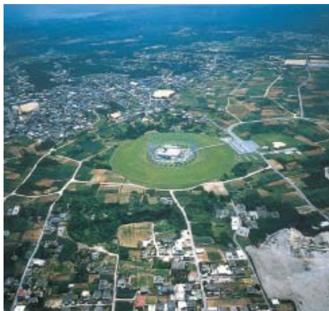
The antenna facilities at Sobe Communication Site (dubbed the "Elephant Cage"), which will be relocated to Camp Hansen.
