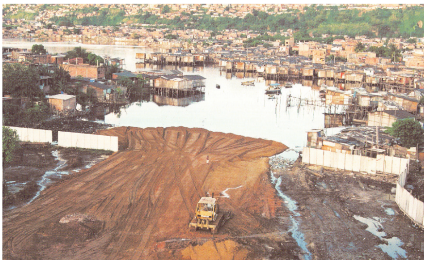
Upgrade in progress in Brazil
