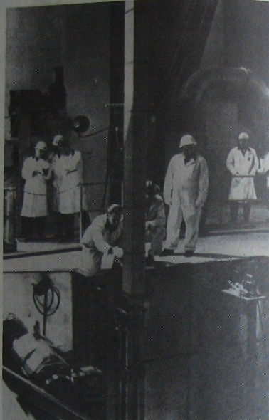
A fuel assembly is lowered into the core of a pressurised water reactor
