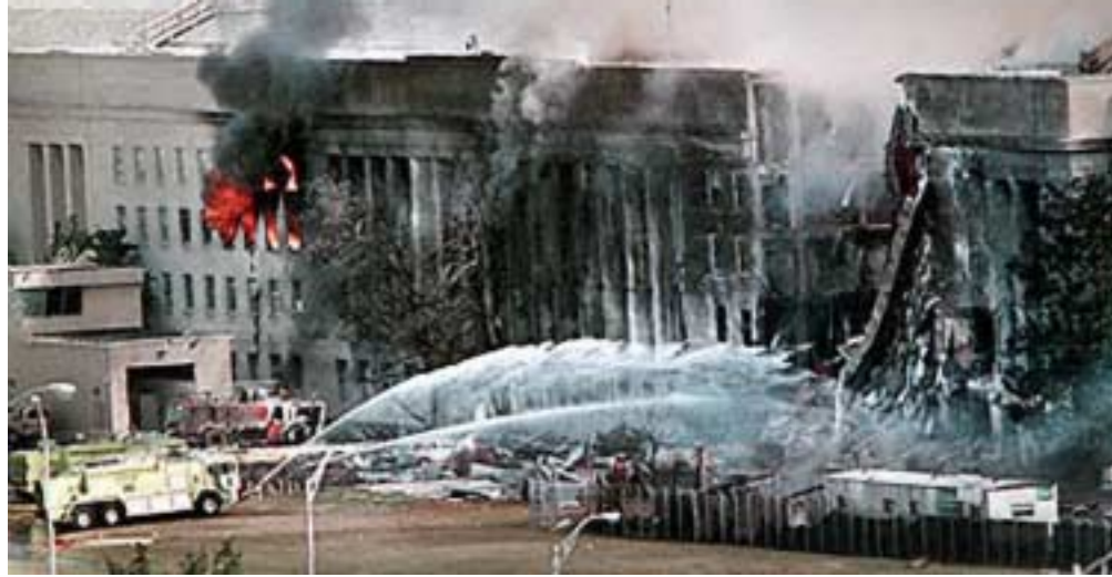
View of external damage.
