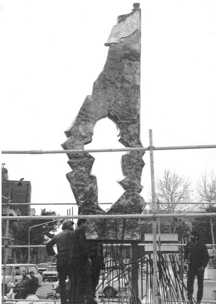
Installation of Monument in Palestine Square, Tehran, March 1986
