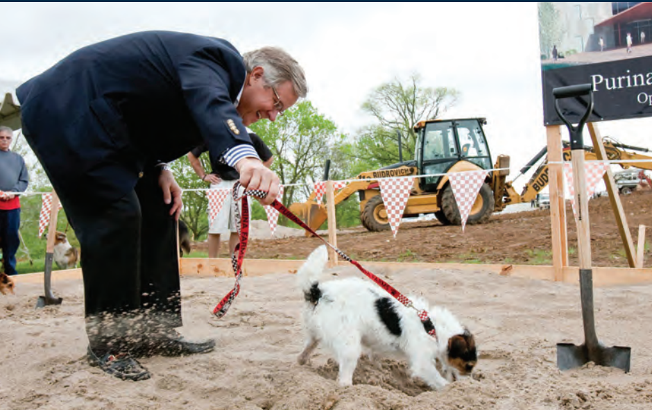
Led by Nestlé Purina President Terence Block, "Chance," a Parson Russell Terrier, helps to break ground on the new $10 million Purina Event Center.
