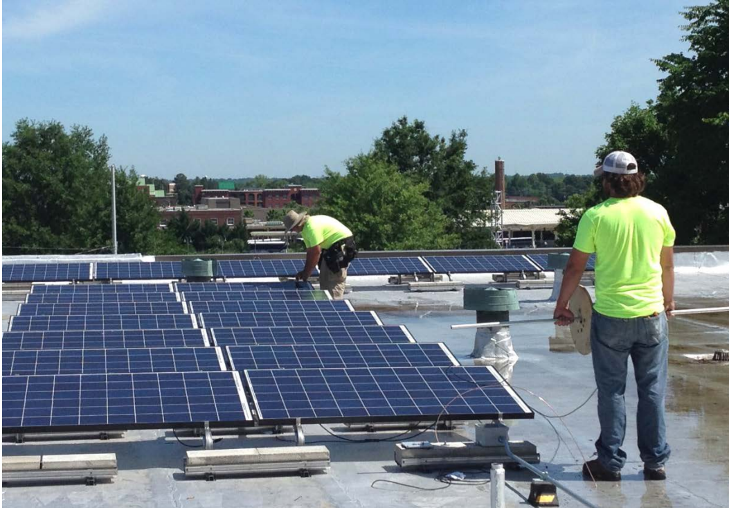
Installation of 5 kW solar photovoltaic system in progress on the rooftop of Faith Community Church, 417 Arlington Street, Greensboro, NC 27406
