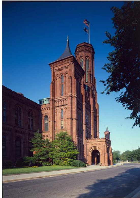
View of the Smithsonian Castle. Image from the National Parks Service Historic American Buildings Survey. Image credit: Jack E. Boucher.
