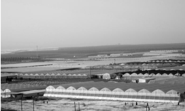
Greenhouses belonging to the illegal settlement of Argarman in the Jordan Valley (Corporate Watch 2010)
