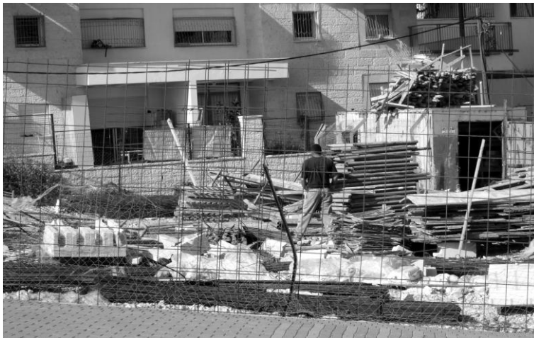
Palestinian Workers on a West Bank settlement construction site (Corporate Watch 2010)
