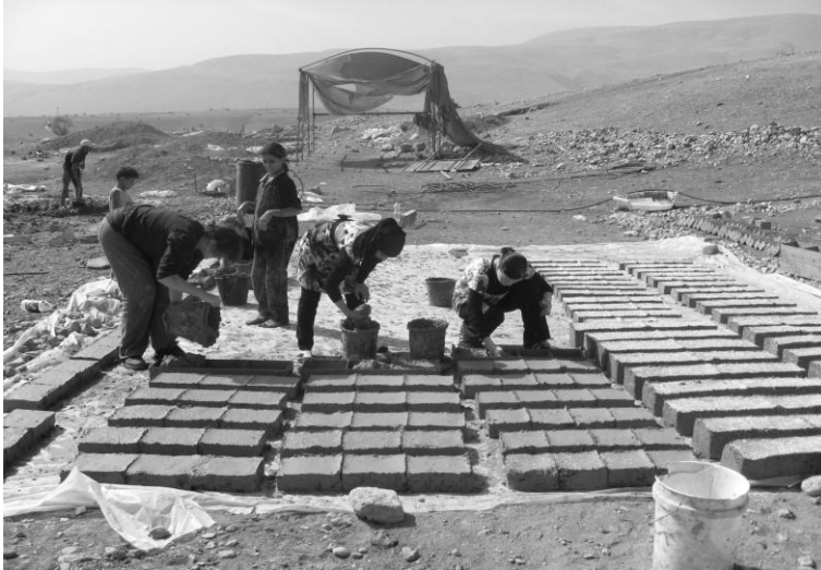
Preparing mud bricks for guerilla building projects in Area C (Brighton Jordan Valley Solidarity 2009)
