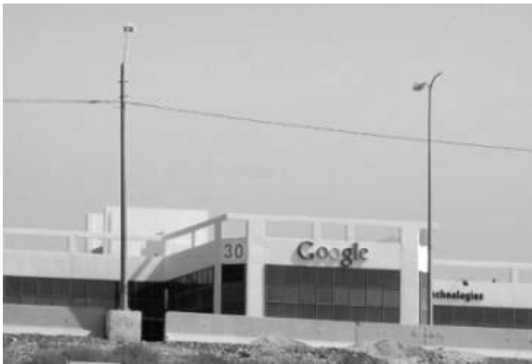
Google's facility in Haifa
