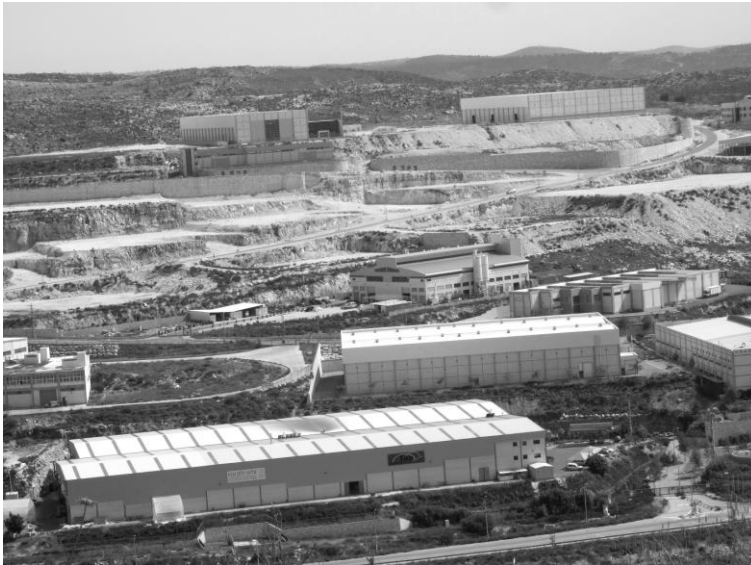
Extension of Ariel West settlement industrial zone under construction (Corporate Watch 2010)
