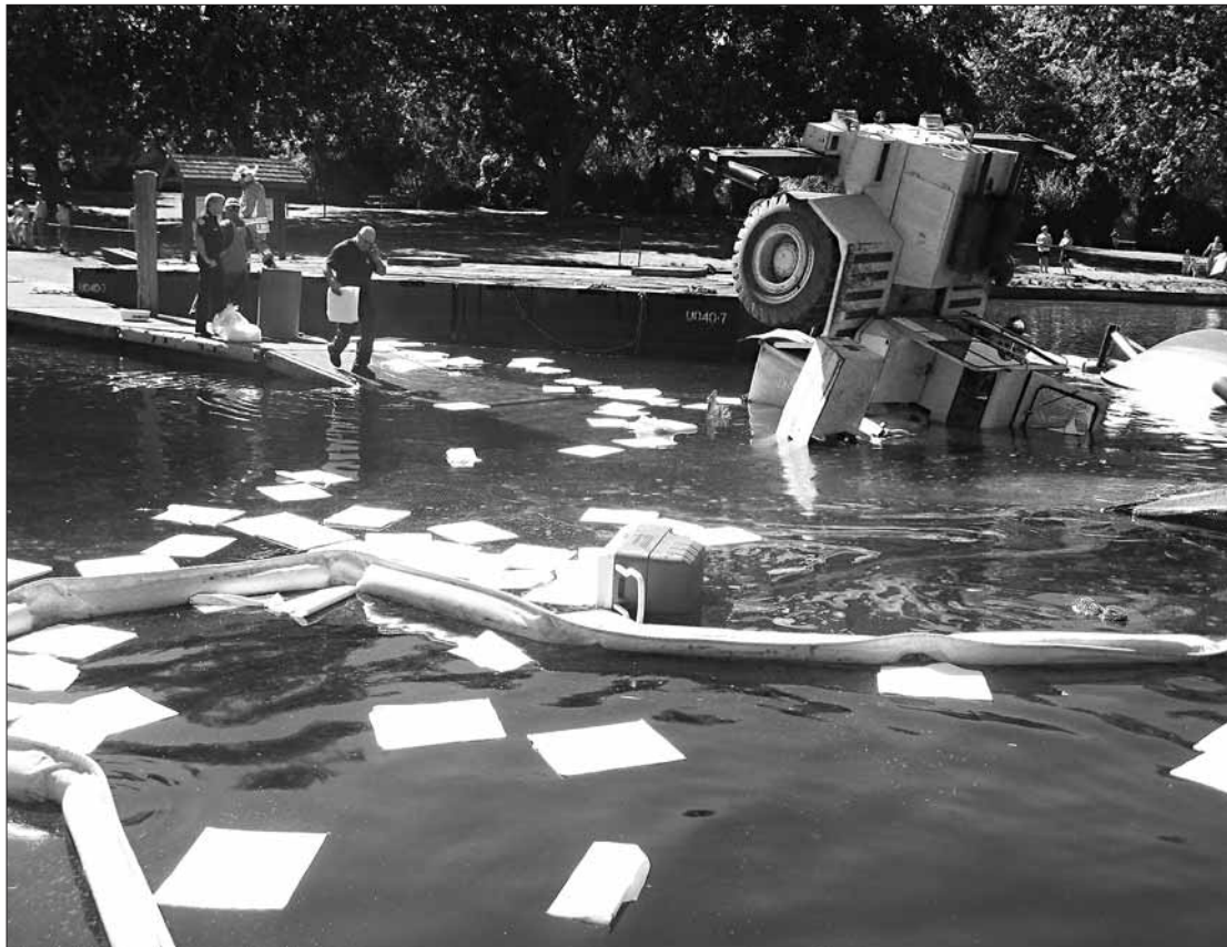
A crane rolled off a barge and into Lake Whatcom at the Bloedel Donovan boat launch late Friday afternoon, overturning an accompanying boat and spilling fuel into the lake in the process. No one was injured in the accident and crane operators quickly deployed absorbent boom and pads to contain and clean up the fuel spill. A larger crane is able to pull the submerged crane from the lake.
